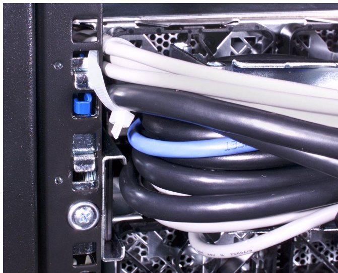
Figure 15. Securing the KVM and SCSI Cables to the Rack
