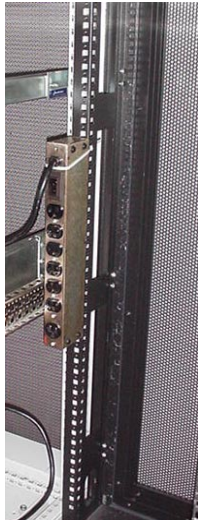
Figure 16: PDUs in a PowerEdge 4210 42U Rack
