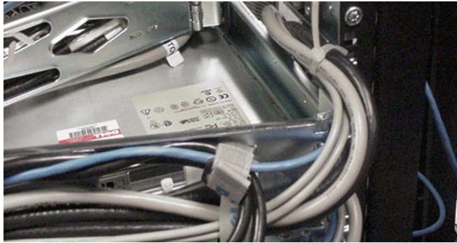
Figure 8: Routing Location for Dell PowerEdge 4210 42U Rack and PowerEdge 2400 24U Racks
