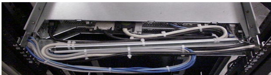
Figure 13: PowerApp 100 System Cabling to 0U Space Through Bracket Cutouts
