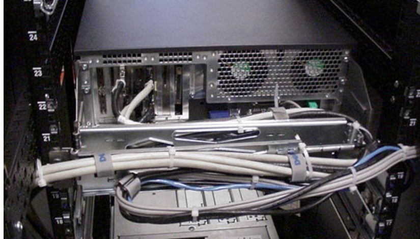
Figure 6: Zip Tying Cables to CMA
